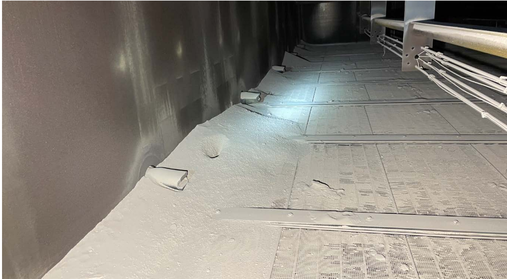
Unit 4 1 st Layer Plugging
