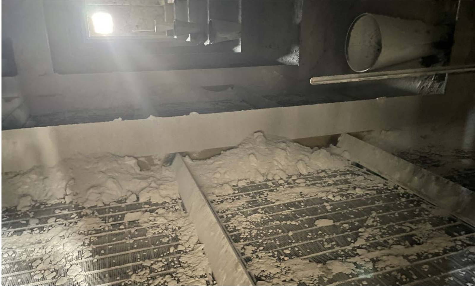
Unit 4 2nd Layer Plugging
