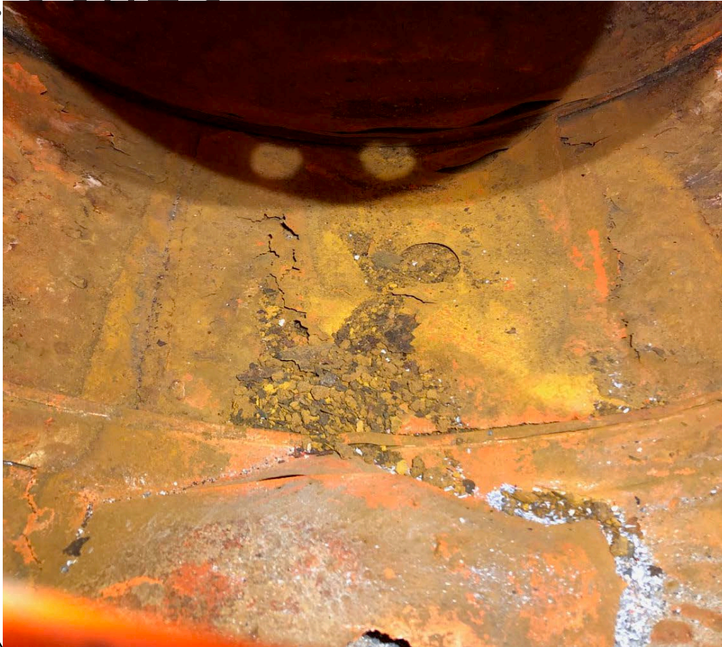
Corrosion from Positive Pressure System
