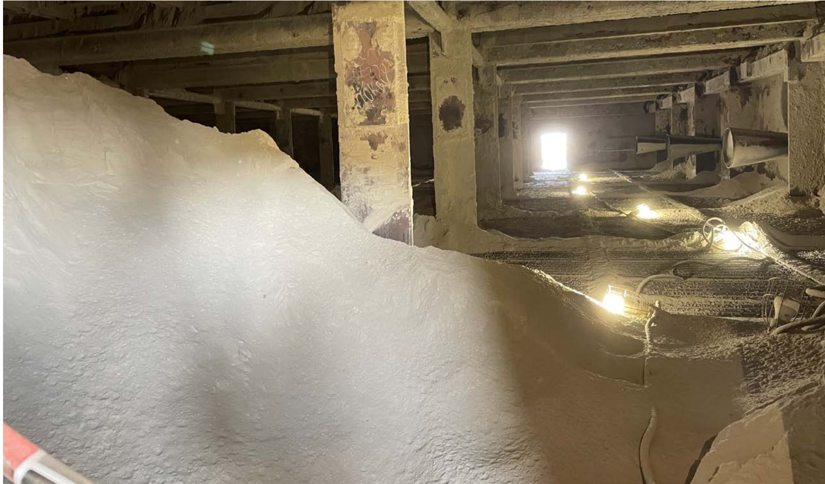
Unit 5 2nd Layer Plugging
